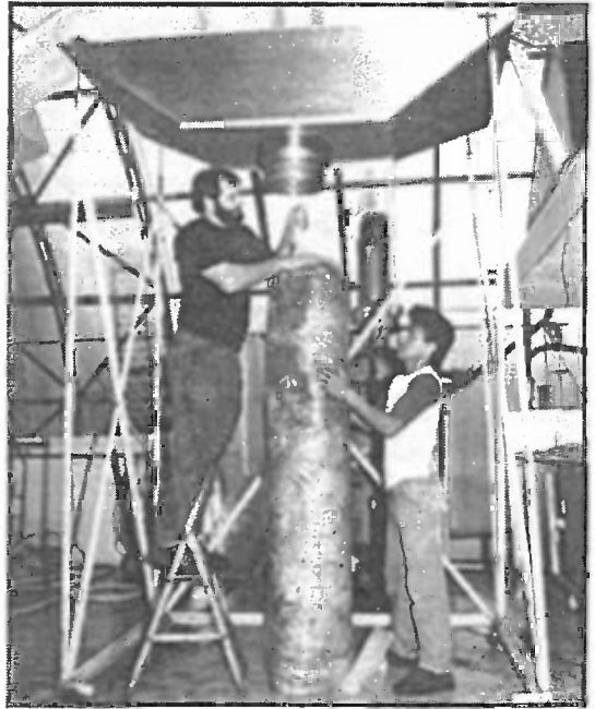
Figure 172 & 173. Once filled, the collar is released and the plastic is tied into a knot.
